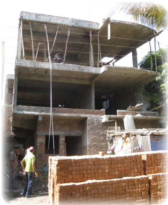
Construction continues on Bhopal residence for philosophy students.
